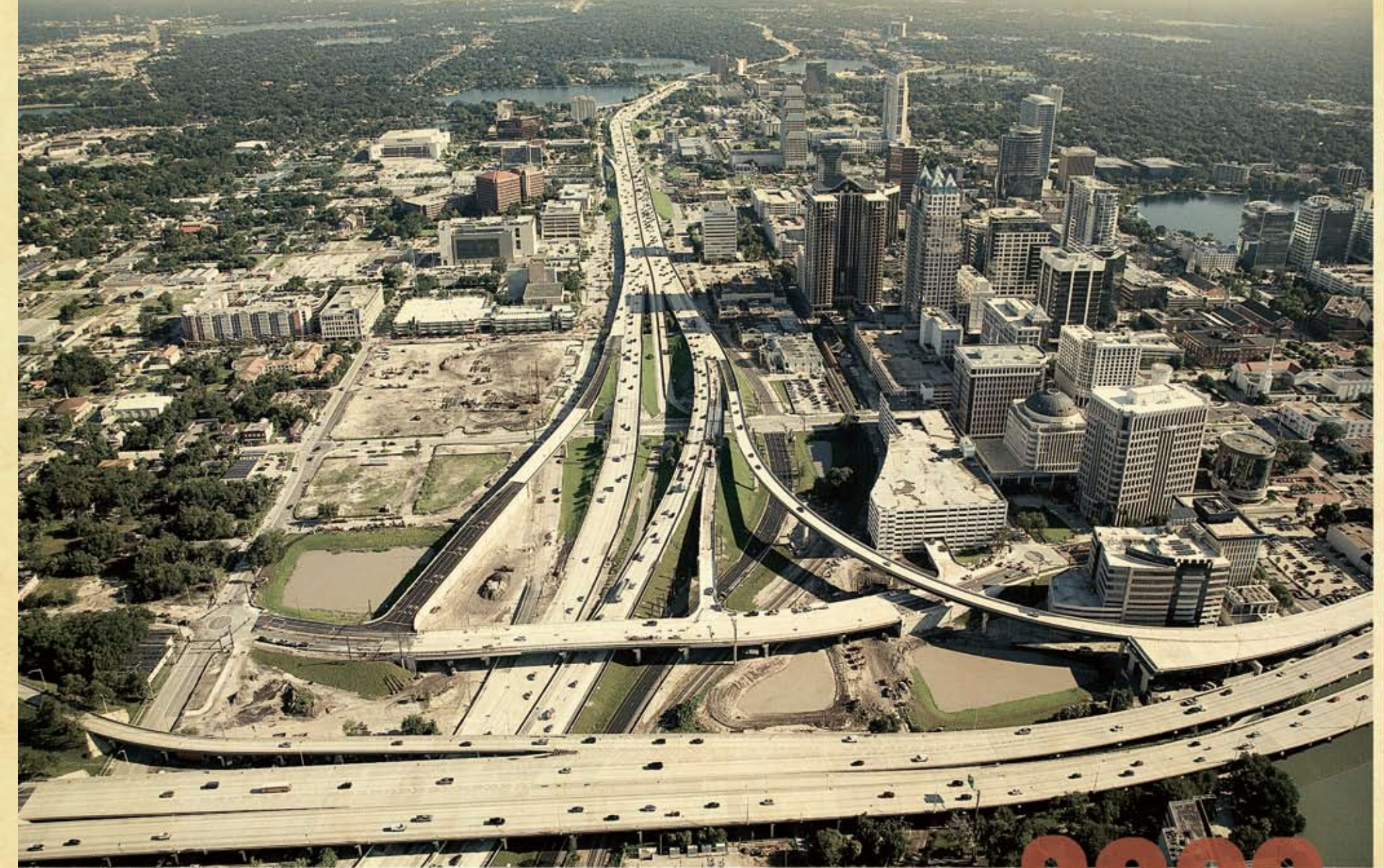
Construction on the interim I-4 and SR 408 interchange nears completion.
