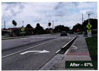
During the initial baseline data collection, drivers were only yielding to pedestrians at this intersection 29% of the time. Since then, Osceola County cleared away the visibility-obstructing bushes in the median and installed a rectangular rapid-flashing beacon, and the average yield rate at this crosswalk has risen to 67%.
