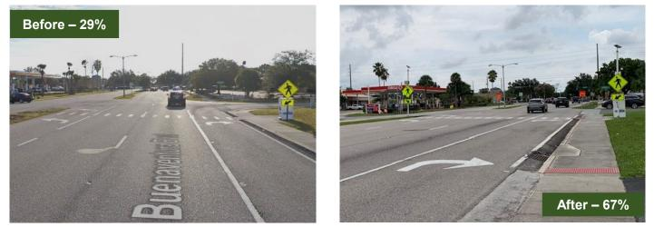
During the initial baseline data collection, drivers were only yielding to pedestrians at this intersection 29% of the time. Since then, Osceola County cleared away the visibility-obstructing bushes in the median and installed a rectangular rapid-flashing beacon, and the average yield rate at this crosswalk has risen to 67%.
