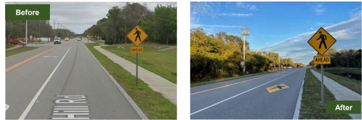
Best Foot Forward has been monitoring this intersection for three years. Toward the end of FY 2022, Seminole County added pedestrian symbols to the road as a preliminary countermeasure. Data collectors have not recorded any measurable improvement in driver yield rate here, likely due to the high speed of traffic. This location is expected to get a pedestrian hybrid beacon in the future to help protect trail users.
