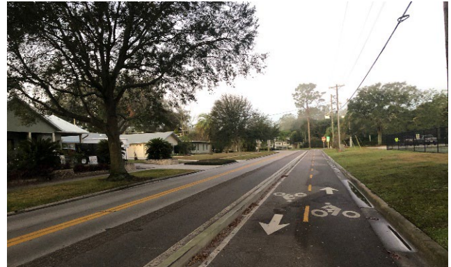
Image 3: Separated Bicycle Facility Example
