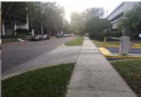
Level sidewalks with short driveway ramps. Image Credit: KAI
