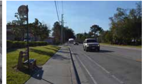
Non-accessible bus stops just west of Thacker Ave
