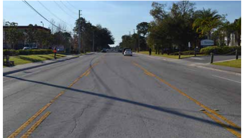
Wide roadway cross section encourages high vehicle speeds
