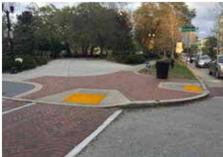
ADA Pedestrian Directional Ramps Photo Credit: KAI
