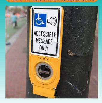
It is necessary that pedestrian facilities be compliant with the Americans with Disabilities Act (ADA), from the width of the facility, to the grade of curb ramps, and the type of materials used. While not an ADA requirement, new signalized intersections should provide audible pedestrian signals (APS) to accommodate pedestrians with visual impairments.
