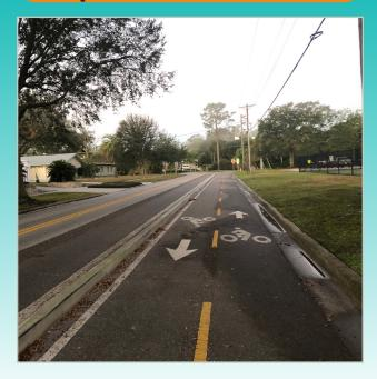
Separated Bike Lanes are similar to Protected Bike Lanes. However, instead of being physically separated from vehicles and pedestrians by vertical delineation, they are separated by horizontal delineation or small, mountable delineation. Separated bike lanes can be one-way or two-way.
