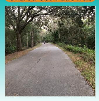
Shared Use Paths are typically separate from the roadway network and provide two-way directional paths for bicyclists, pedestrians, and other non-motorized users. According to the Florida Design Manual (FDM) 224, shared use paths should meet the following widths:
