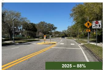
This crosswalk was originally monitored by the Best Foot Forward program from 2013 to 2018, with a final driver yield rate average of **49%**. By 2023, this crosswalk had been relocated slightly west (now a midblock) with a Rectangular Rapid Flashing Beacon installed. Data collection in 2025 shows an average of **88%** of drivers yielding to pedestrians here.
