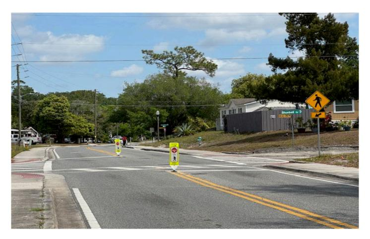
Located in a neighborhood, this crosswalk has continued its improvement from a driver yield rate average of just 16% in 2023, to 47% in 2024, and now 63% in 2025. This follows the installation of in-street signage and stop bars in 2024 as well as two crosswalk enforcements over the same time window from the Casselberry Police Department, resulting in 26 warnings and citations to drivers who failed to yield to pedestrians.
