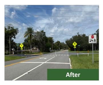
Located right off the Seminole Wekiva Trail, Best Foot Forward data collectors recently recorded a **70**% driver yield rate at this crosswalk after installment of in-street flex posts, new fluorescent double-sided yellow pedestrian signage, and in-road pedestrian markings.
