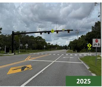
A Pedestrian Hybrid Beacon (PHB) was installed at this trail crossing in the summer of 2025, along with "Stop Here for Pedestrians" signs, stop bar markings, and delineated high-visibility ladder striping.
