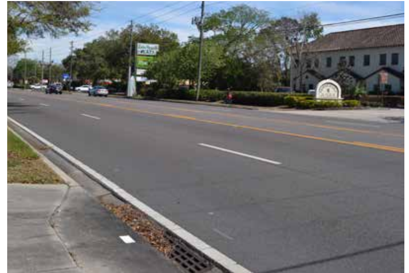
The wide roadway cross section encourages high vehicle speeds
