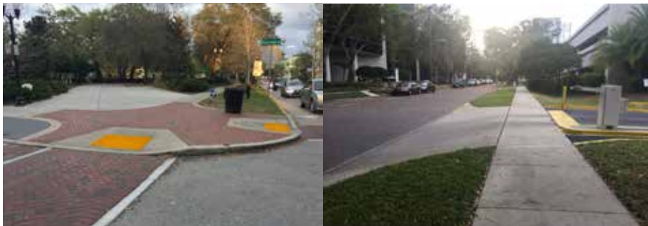
Right-sized curb radius and ADA Pedestrian Directional Ramps Photo Credit: KAI
