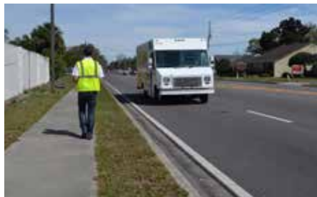
High vehicle speeds and a narrow grass strip cause uncomfortable pedestrian environment
