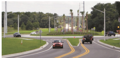
CR 561 and CR 455 Roundabout (Lake County) - Through an FDOT Local Agency Program (LAP) project, Lake County recently constructed a roundabout at CR 561 and CR 455. The existing stop-controlled intersection had a 61% higher crash rate than the Florida state average. There have been no reported crashes since the roundabout opened in 2015.
