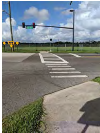
Figure 44. Faded Crosswalk Issue
