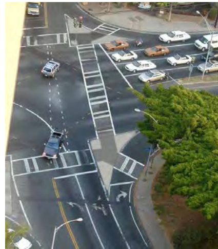
Channelized Right-Turn Lane with Enhanced Pedestrian Crossing
