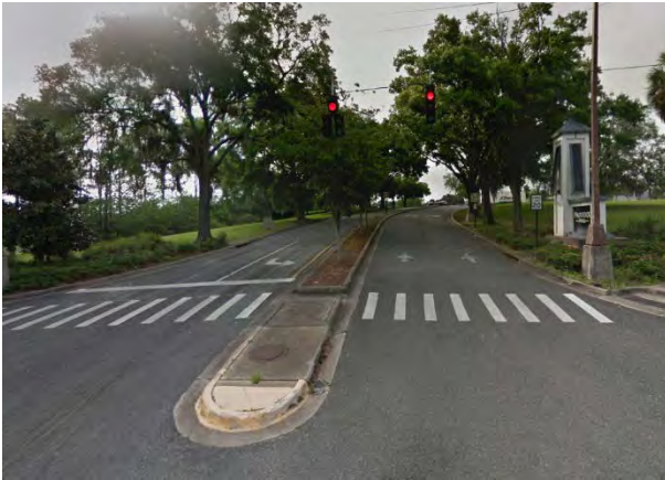
No Sidewalks Provided for Mall Access (pedestrians must walk in road)
