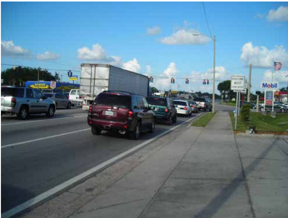
Figure 18 Colonial Drive at John Young Parkway, looking east
