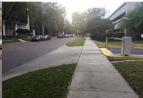
Level sidewalks with short driveway ramps. Image Credit: KAI
