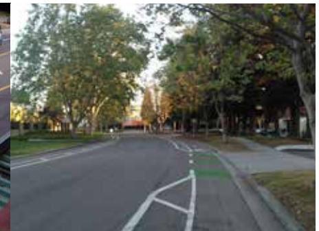
Use of green bike lane at driveways Photo Credit: Safe Mountain View Blog
