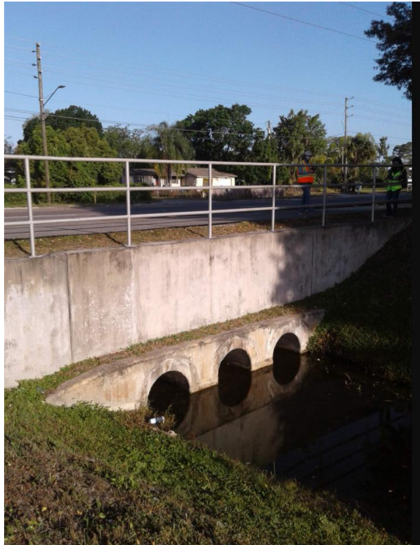
Figure 20 | Triple 36-inch Cross Drain
