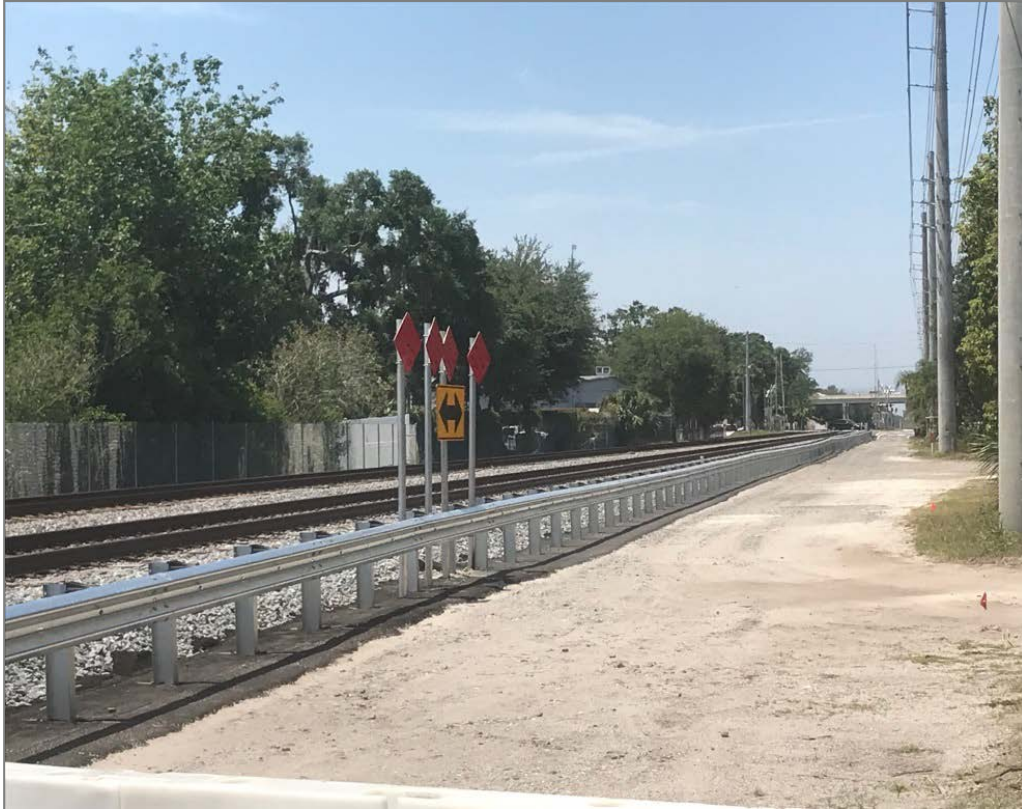
Added guardrail along Clay Street
